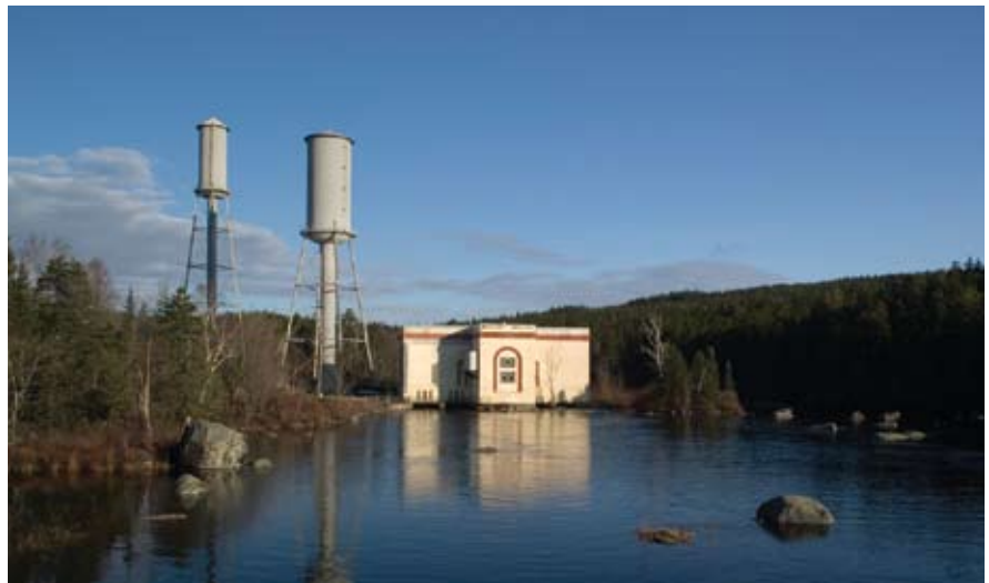
St. Margerets Bay Hydro
