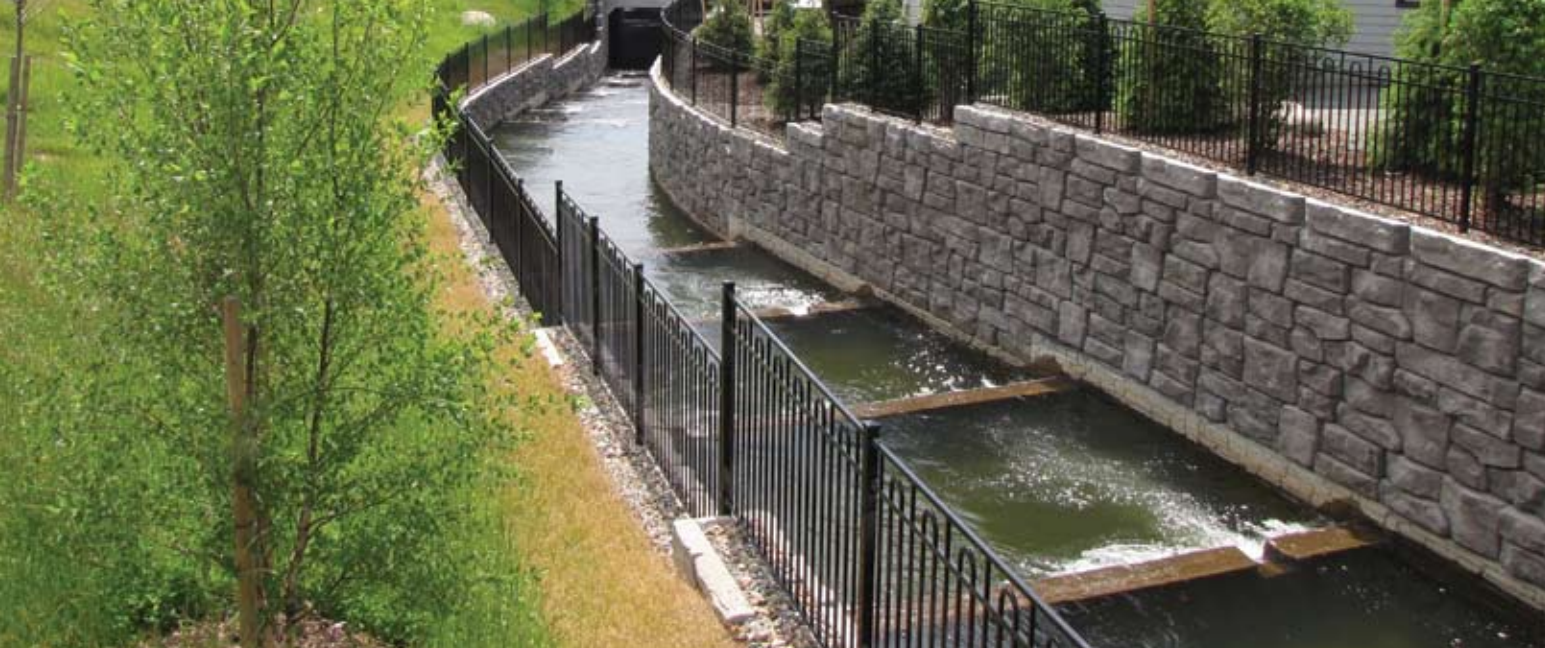
Sullivan's Pond Stormwater System Renewal
