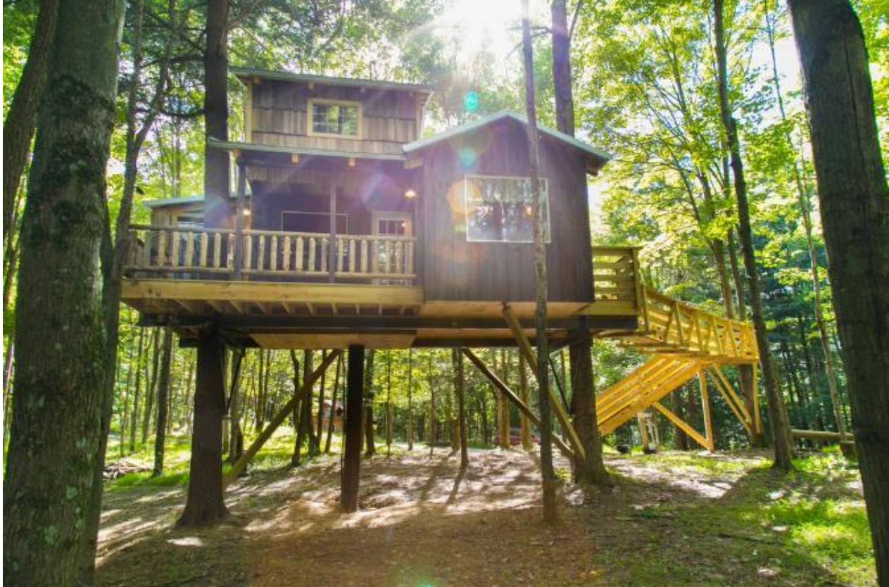
Figure 19: Creative Camping Cabins – The Mohicans, Ohio
