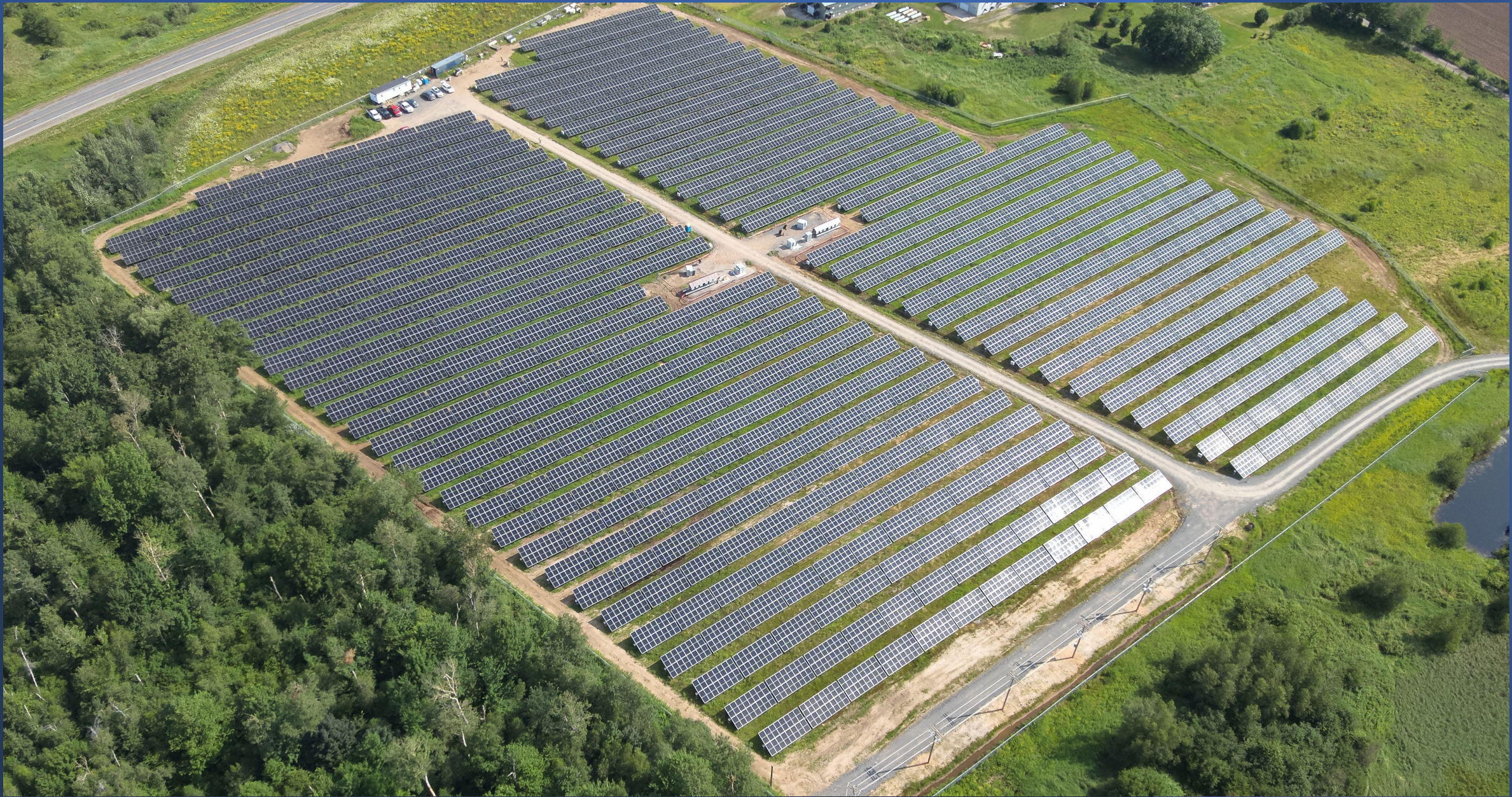
Town of Berwick 3.45MW Solar Garden
