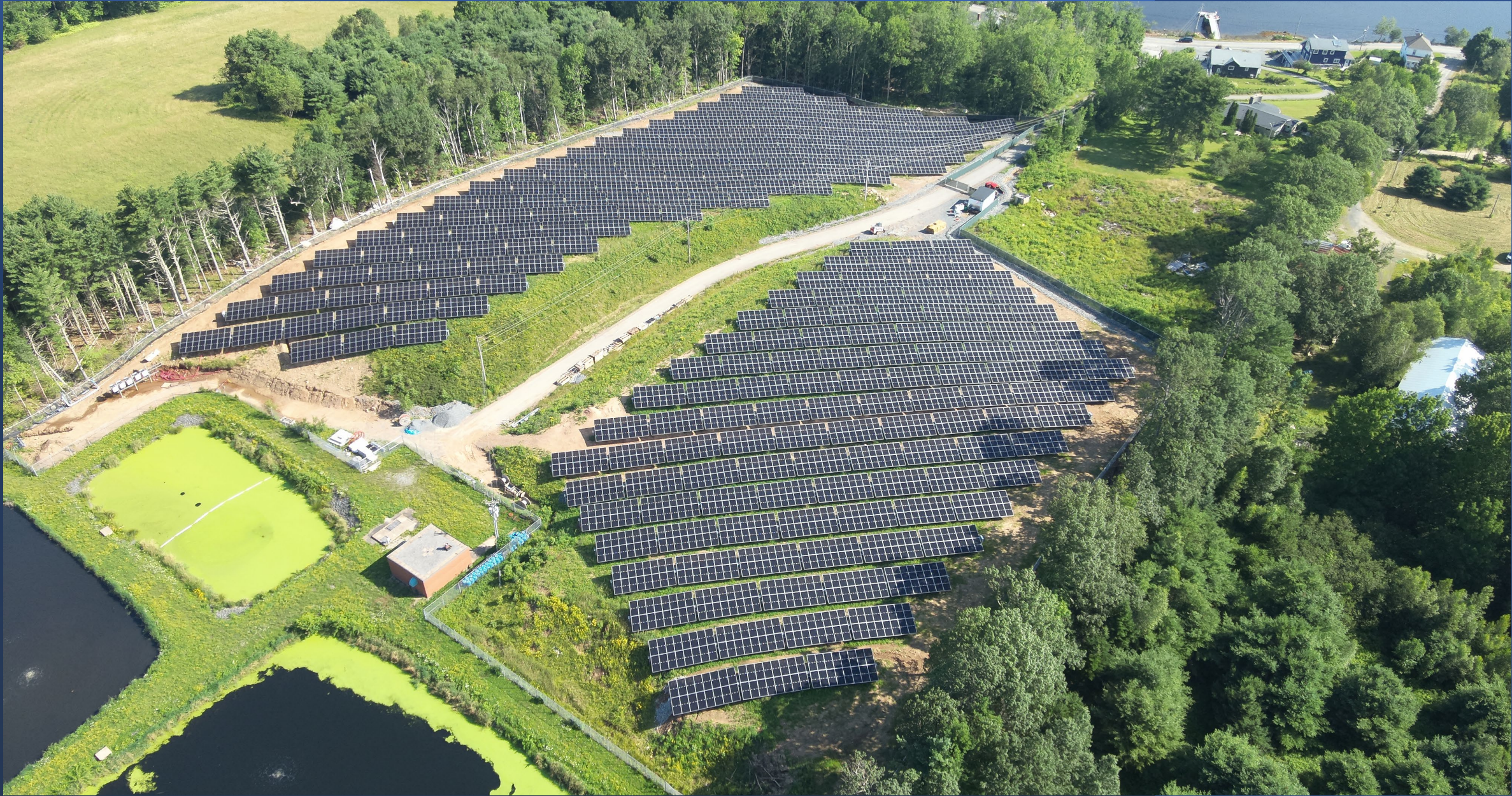
Town of Mahone Bay 1.5 MW Solar Garden
