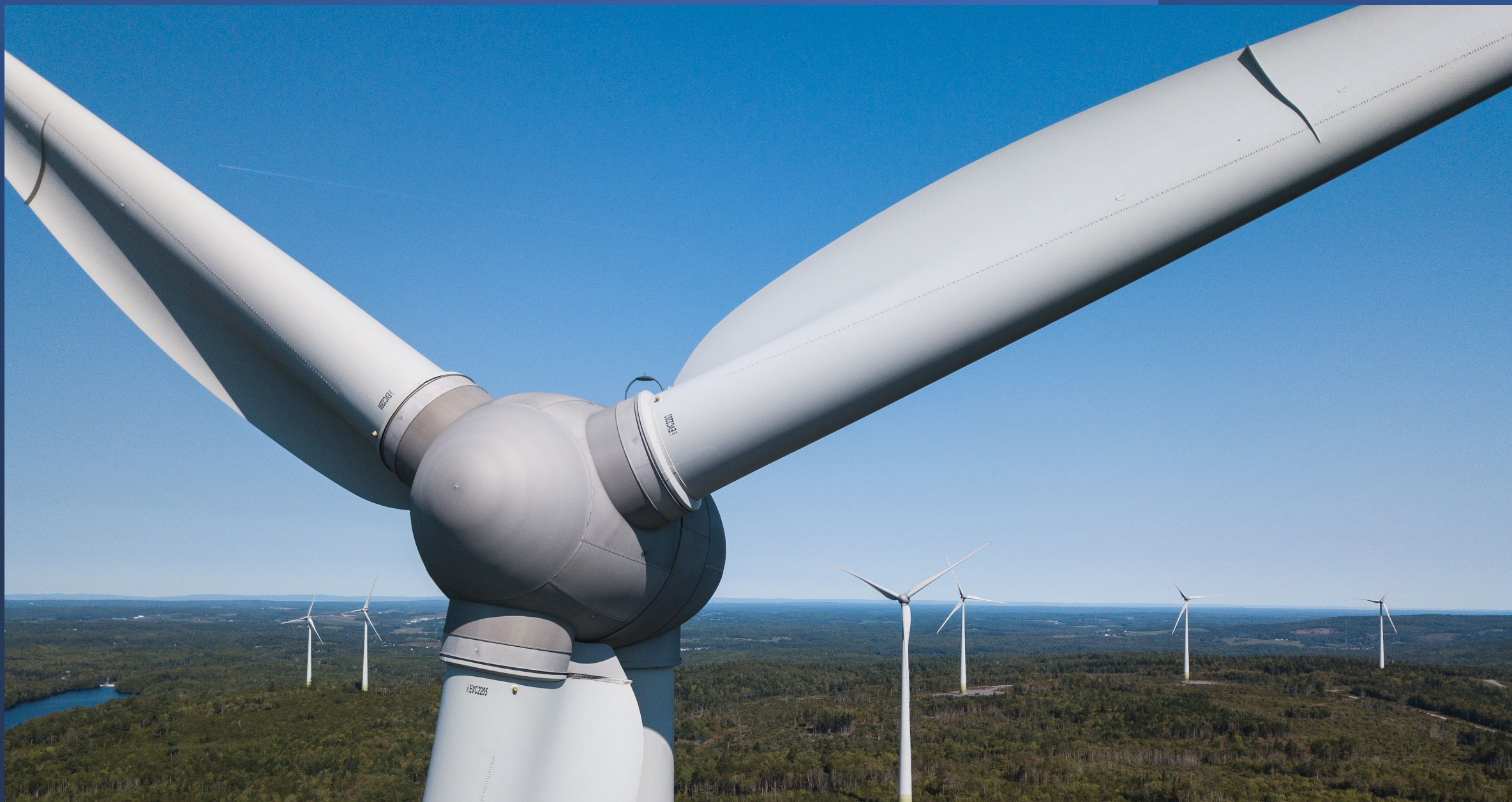
Ellershouse Wind Farm 23.5 MW
