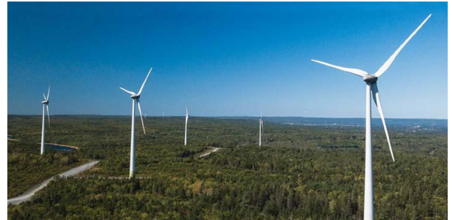
Ellershouse Windfarm (Source: AREA)
