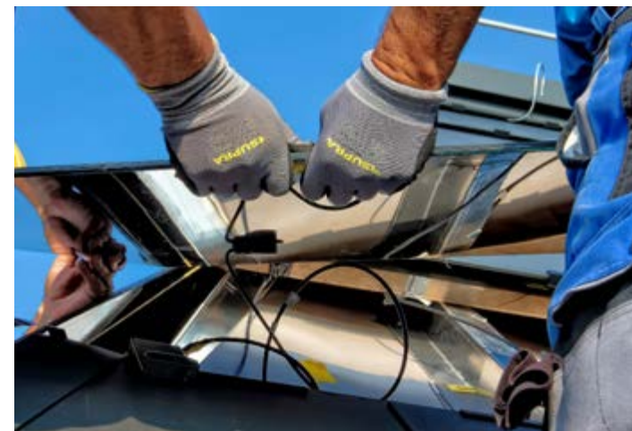
Panel Construction (Source: UnSplash)
