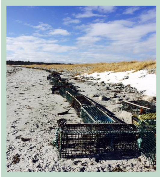
Left-hand photo: Newly installed lobster traps have yet to be covered in sand and marram grass. Right-hand photo: With time, sand and marram grass begin to cover the lobster traps put along the revetment.
